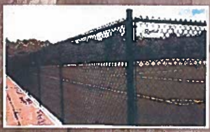
The East Fence is Typical black 6' high chain-link fence.
