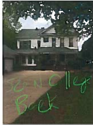
Rear of main structure, Jackson Street side.
