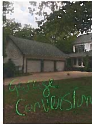
On Jackson Street side, to be converted.
